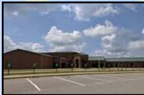
Terrell County SBHC
